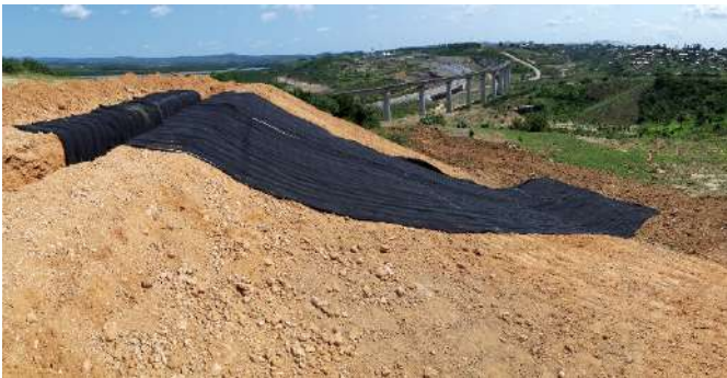
Deployment in slopes and anchor trenches
