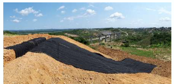
Unrolling the SOMTUBE FTF in the slope and anchor trench
