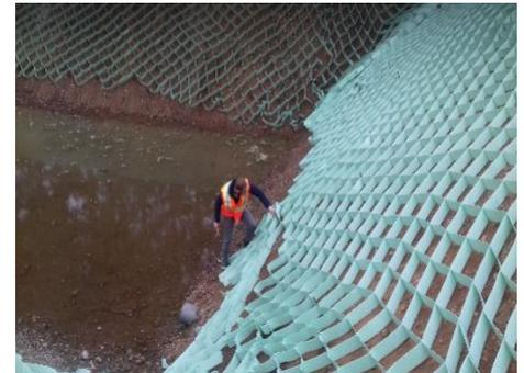
Adjustment and installation of anchor pegs according to design calculations
