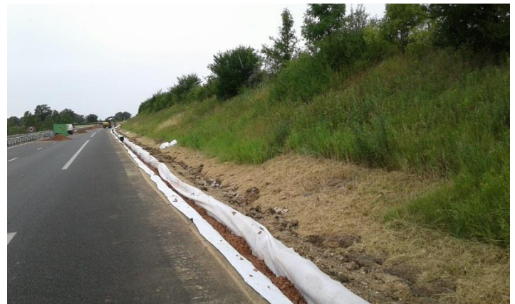
Installation inside the trench and backfilling
