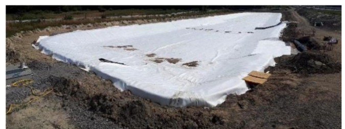
Installation of the puncture-resistant geotextile
