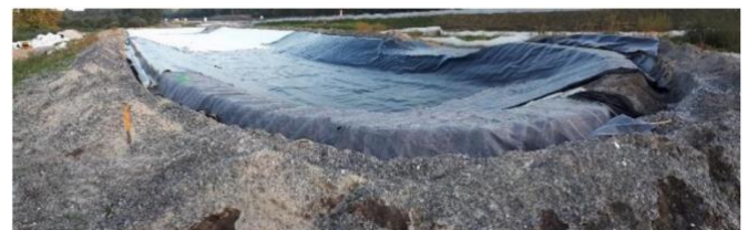
Installation and welding of the geomembrane on the DRAINTUBE
