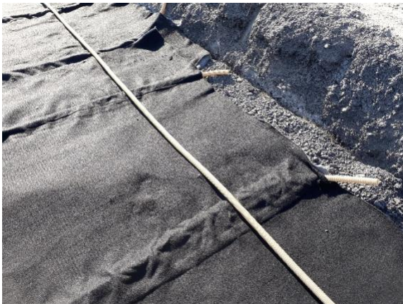
Installation of the \phi 25 -mm drain
