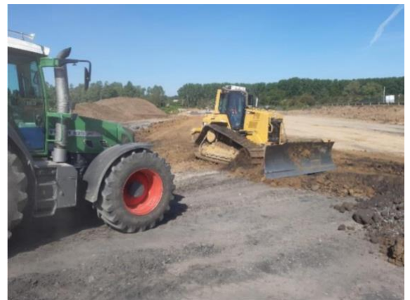
Water-saturated loam soil of the site, prepared to host SOMTUBE FTF
