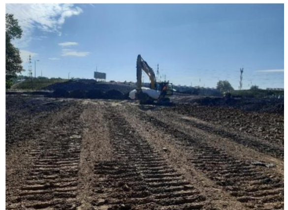
Handling of SOMTUBE FTF on site
