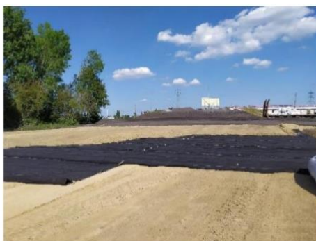
Connection to the peripheral ditch, backfilling and compaction
