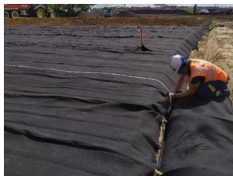
Connection to the peripheral ditch, backfilling and compaction
