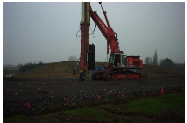
Installation of vertical drains
