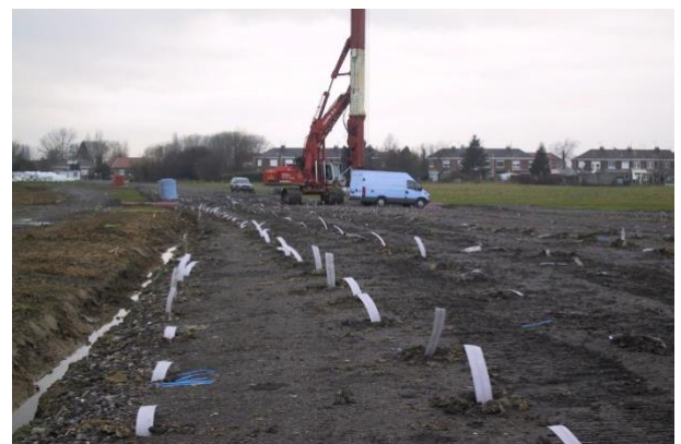
Vertical drains on the platform
