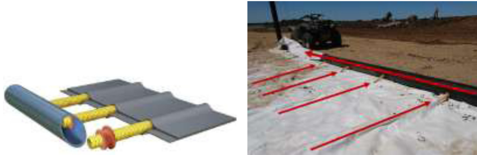
Fig. 1. Multi-linear drainage geocomposite connection scheme on the left and connections configurations on site on the right.
