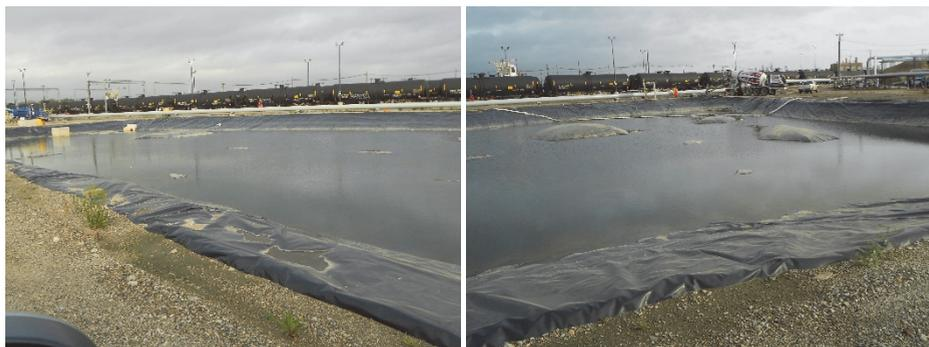
**Fig. 9.** Geomembrane uplifts in Pond 1.
