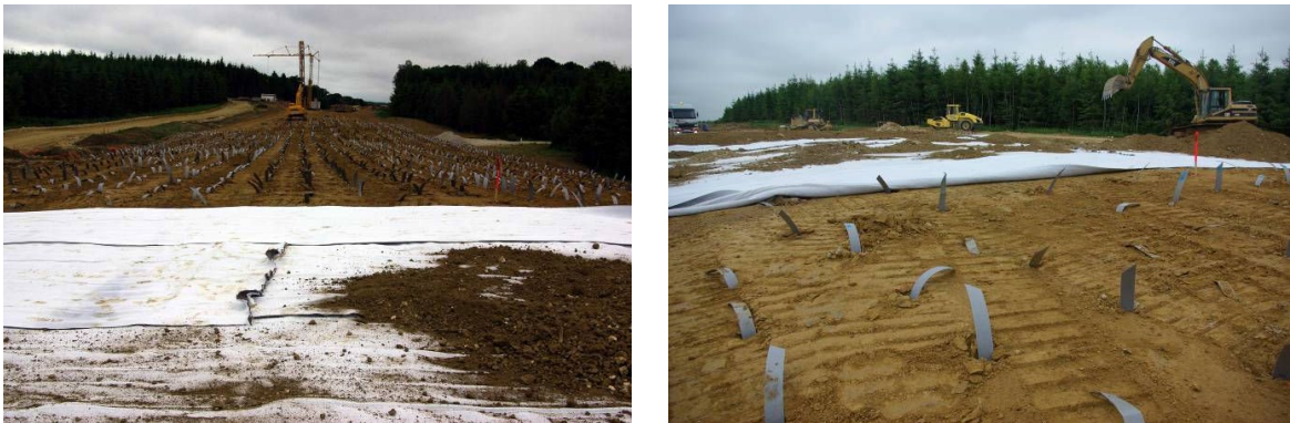
Figure 5 and 6. Installation of the Drain Tube
