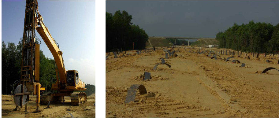
Figure 3 and 4. Installation of the vertical wick drains.
