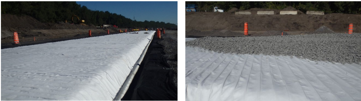
Figure 14 and 15. Installation of the geocomposite and backfilling with ballast
