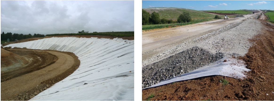
Figure 8 and 9. Drainage mask construction with drainage geocomposite
