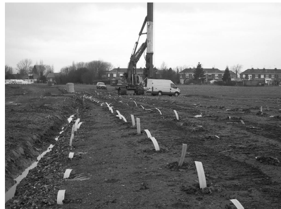
Figure 1 Installation of the geosynthetic vertical drains
