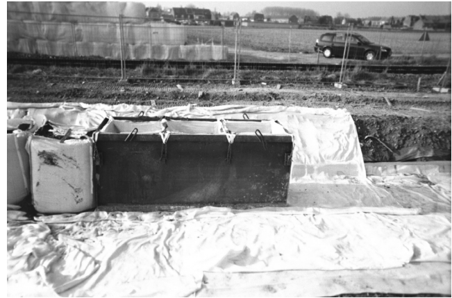
Figure 8 View of the big-bags and removable shuttering
