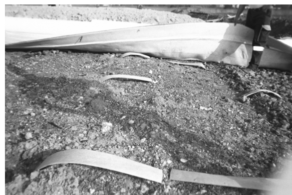
Figure 2 Horizontal drainage combined with the vertical drains
