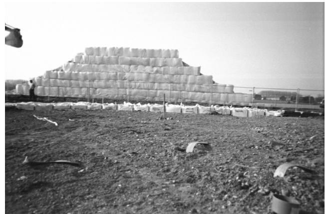
Figure 9 Final aspect of the reinforced walls
