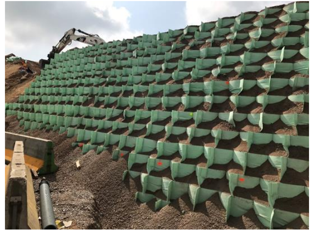
Figure 14. Elevation of the retaining structure
