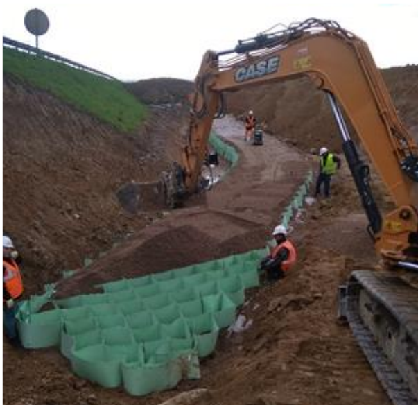
Figure 13. Backfilling and compaction
