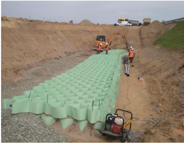
Figure 12. Geocells deployment
