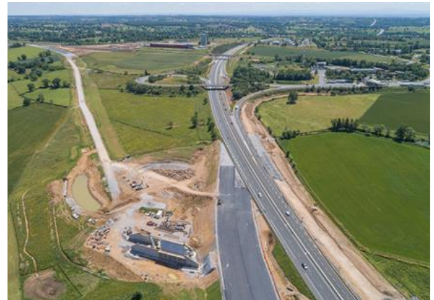
Figure 4. Aerial view of the bypass (© Philippe Busser | XXI communication | APRR)
