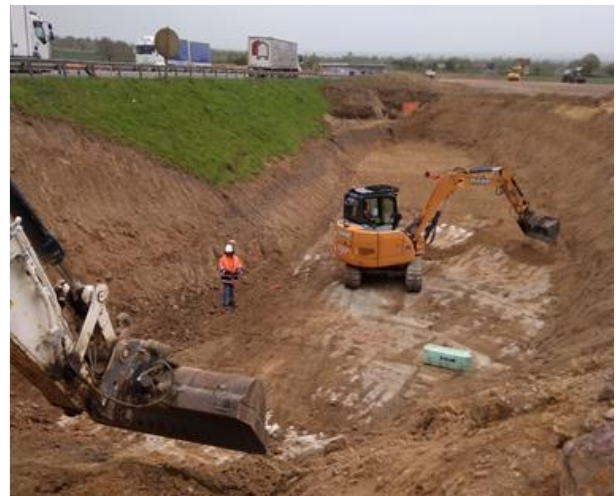
Figure 11. Excavation of the subgrade
