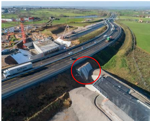
Figure 2. North structure (La Montagne source)
