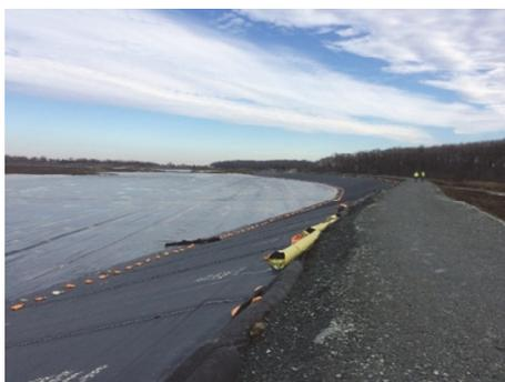
**Fig. 6.** Site photo of deployed geotextile.
