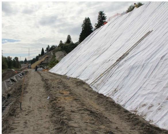
Figure 7. Installation of the DTPDG
