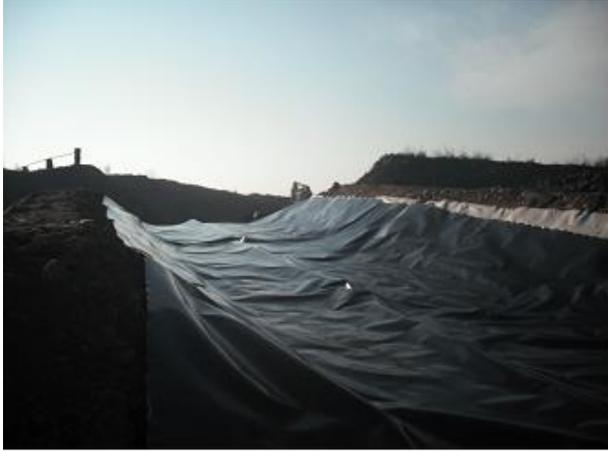
Figure 5: Geomembrane installation
