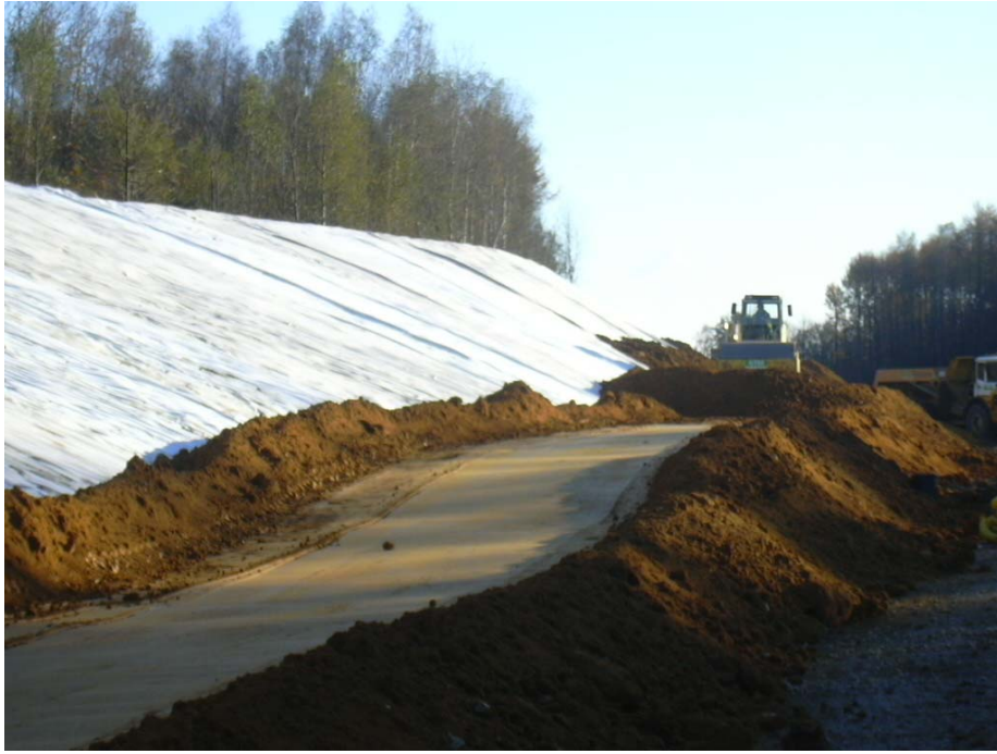
Photo 7. Filling, resurfacing and under-steeping the slope embankment.
