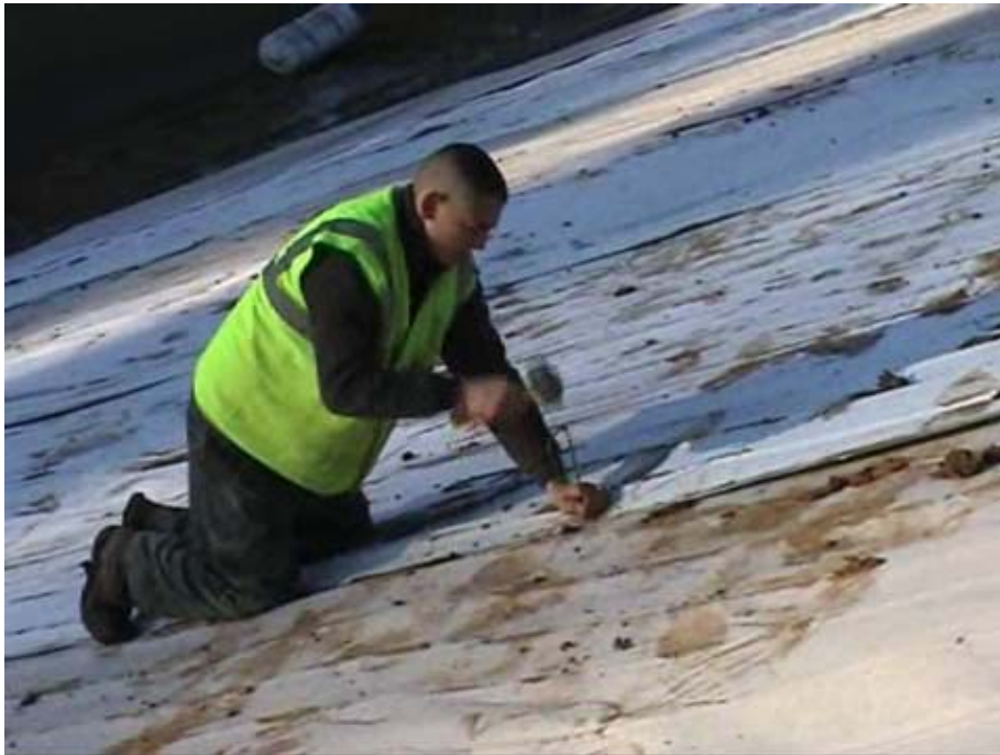
Photo 4. Géocomposite SOMTUBE FTF fixation on the slope
