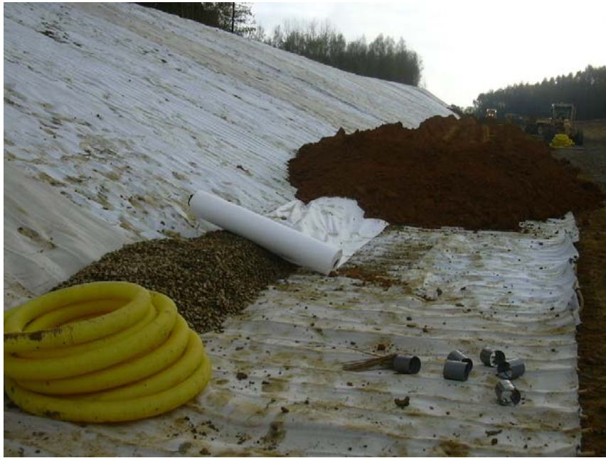
Photo 5. Geocomposite SOMTUBE FTF connection to the collector drain
