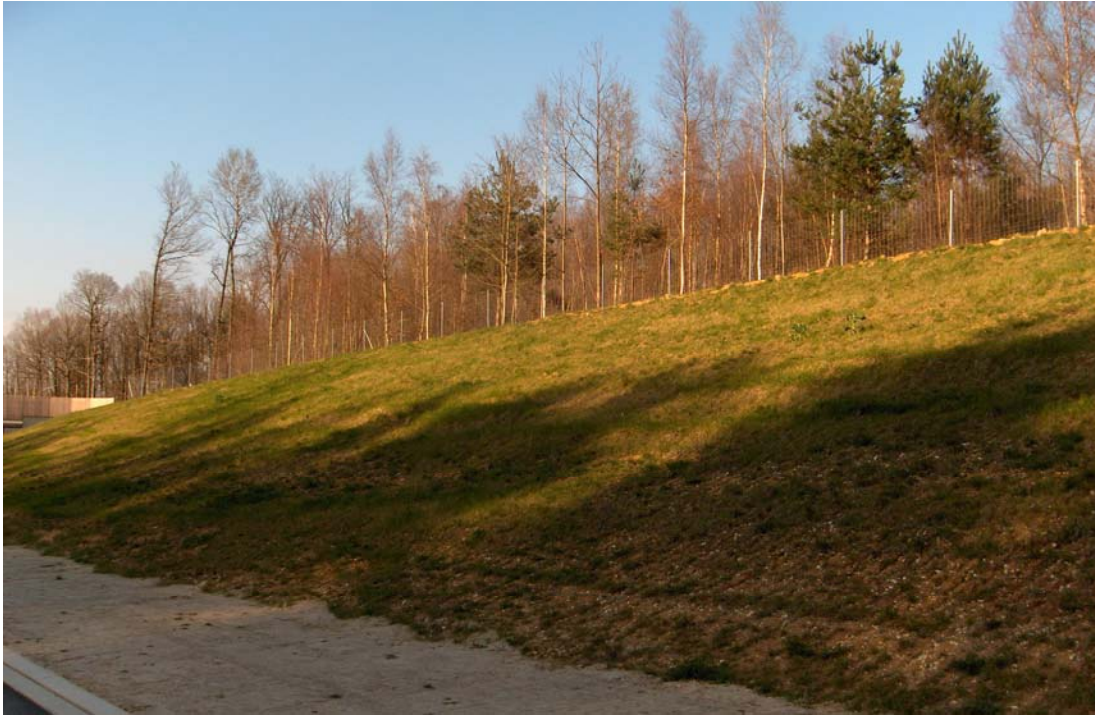
Photo 9. Vegetalisation and intégration of the cut slope in the landscape
