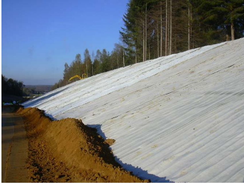
Photo 3. Géocomposite SOMTUBE FTF unrolling
