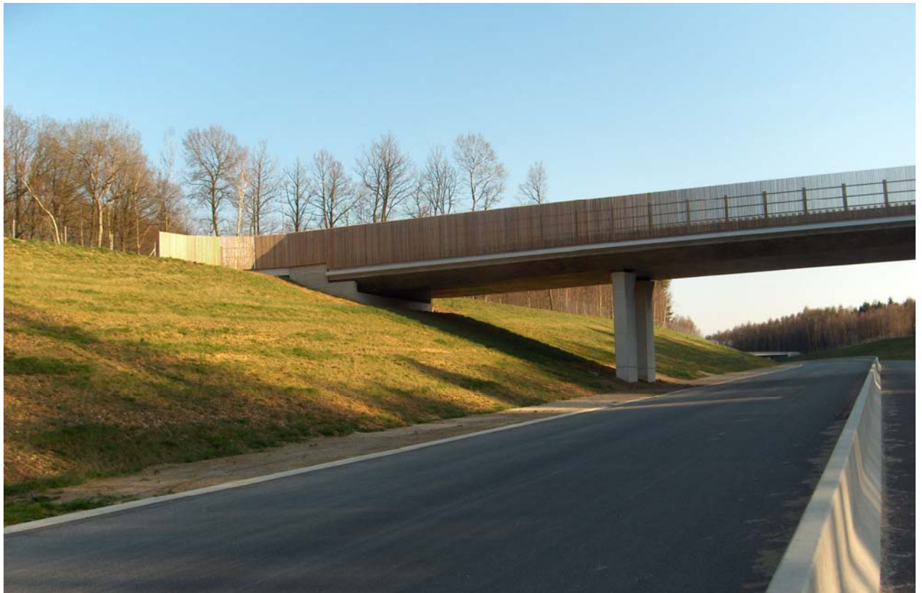
Photo 8. Completion of the cut slope
