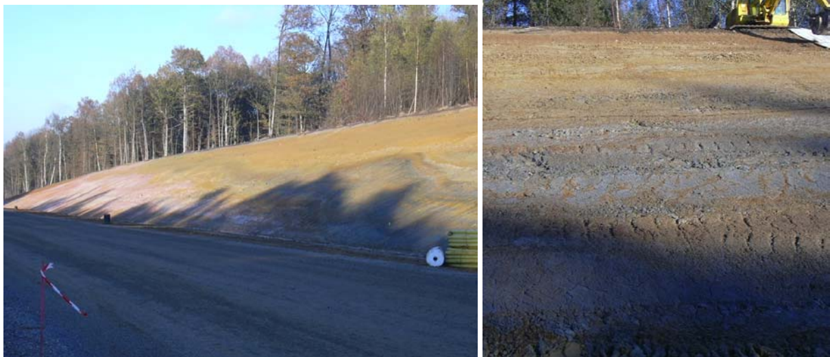
Photos 1 &amp; 2. View of clearance D5 after earth moving work
