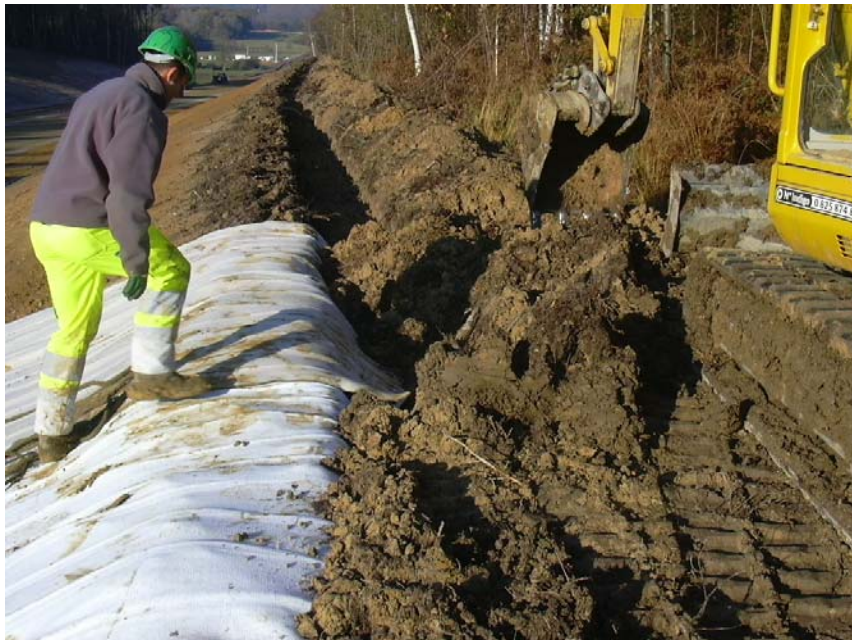
Photo 6. Mechanical fastening at the summit with anchoring.
