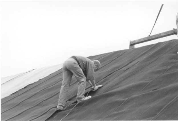
Figure 14. Covering and fastening of sheets.
