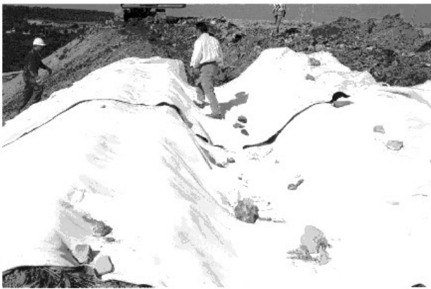
Figure 5. Anchor trench
