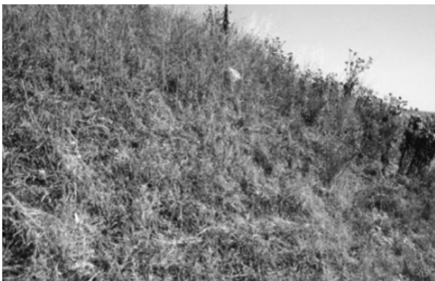
Figure 6. State of section n° 1 over a year later.
