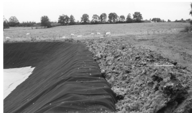
Figure 13. Fastening of a geocomposite drainage layer at the head of the embankment
